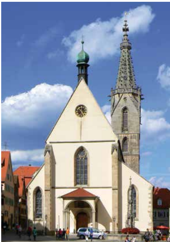
Dom St. Martin, Rottenburg/Neckar
