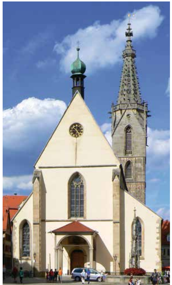
Dom St. Martin, Rottenburg/Neckar
